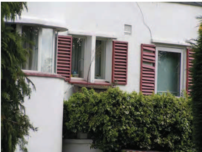
Picture 4.85 Original shutters on number 4 Kerry Avenue
