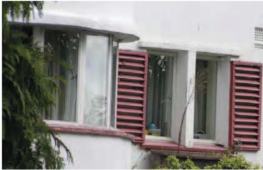
Picture 4.80 Vertical emphasis of Crittall windows along Kerry Avenue, at 4 Kerry Avenue, and right at 5 Kerry Avenue
