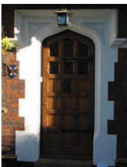
Picture 6.75 Pointed, heavy timber front door with good Tudor Revival doorcase detail
