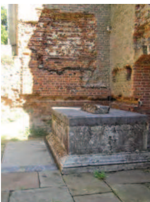
Picture 3.29 Memorial within the Old Stanmore Church
