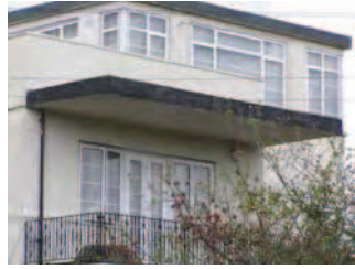
Picture 4.48 First floor balcony to 8 Valencia Road
