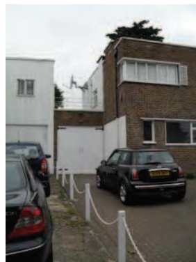
Picture 4.56 Original sundeck feature above side garage of 3 Kerry Avenue
