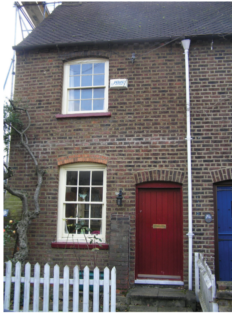
Picture 3.5 29 Middle Road, Harrow on the Hill
