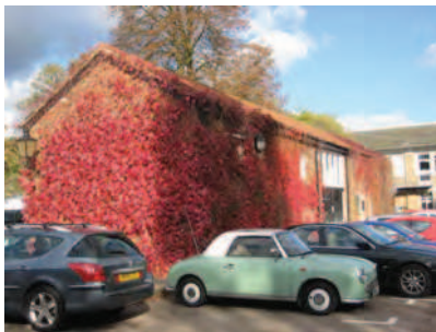
Picture 6.47 Simple, brick design with pitched roof and large wagon doors
