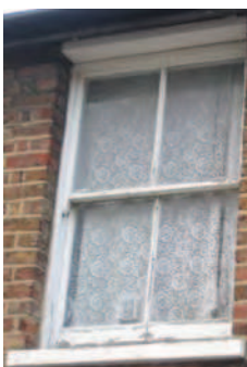
Picture 5.48 The original two over two pane timber sash window on the first floor of the Whitchurch Lane terrace
