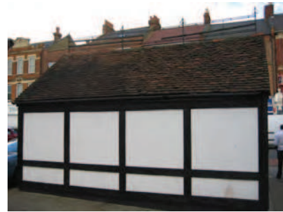
Picture 5.54 Rear of the positive unlisted no. 103 High Street, Edgware
