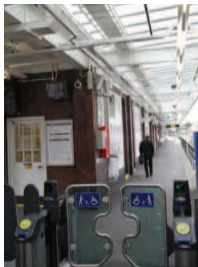
Picture 4.73 Partly original canopy over the platform of Stanmore Station
