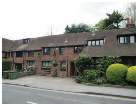
Picture 3.7 Grade II listed Tithe Barn, Old Church Lane
