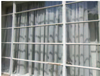
Picture 4.76 Crittall windows that use delicate metal glazing bars to create prominent horizontal panes are typical of those on Valencia Road
