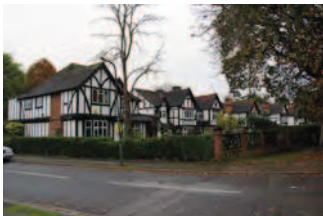
Picture 6.62 Facing the Basin, Canons Drive
