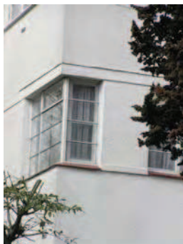
Picture 4.78 Crittall windows sometimes follow the sharp corner of a building to emphasise the strong geometrical forms as above, and in the picture right, on 2 Valencia Road
