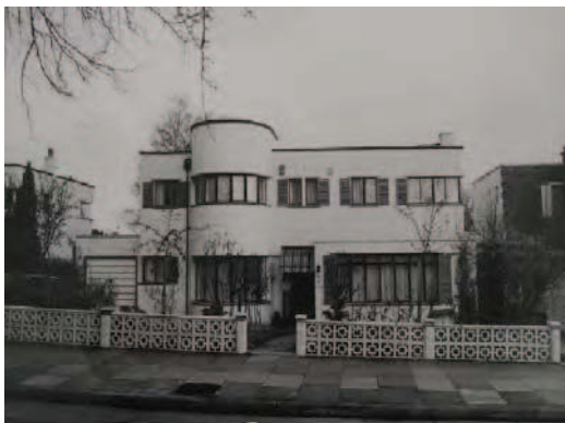
Picture 4.59 Number 4 Kerry Avenue before some of the modern alterations to the building (date of the photo unknown). Source: Local history library
