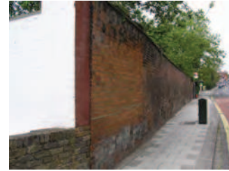
Picture 2.5 Locally listed historic brick wall fronting public highway, lower reaches of Stanmore Hill
