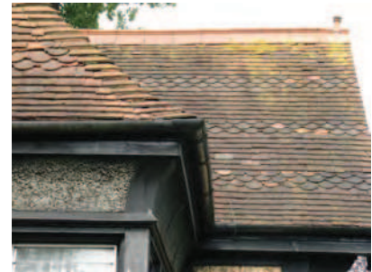
Picture 3.39 Good decorative tile roof
