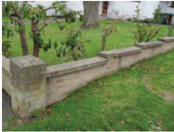
Picture 4.96 Original low boundary treatment to 5 Kerry Avenue of Dunbrik, typical of those original boundary treatments within the Conservation Area
