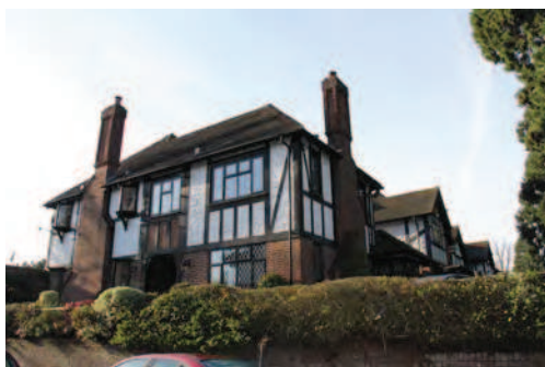
Picture 6.72 Prominent, tall chimneys
