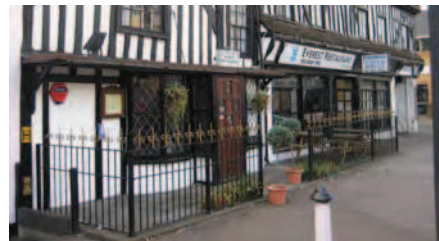
Picture 5.74 Front boundary to nos. 97-99 High Street, Edgware partially obscuring the frontage of the building behind
