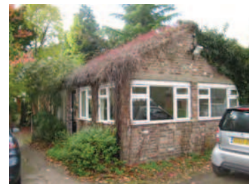
Picture 6.48 Simple single storey brick building
