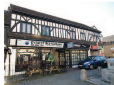
Picture 5.41 No. 97-101 High Street - attractive Tudor style timber framing
