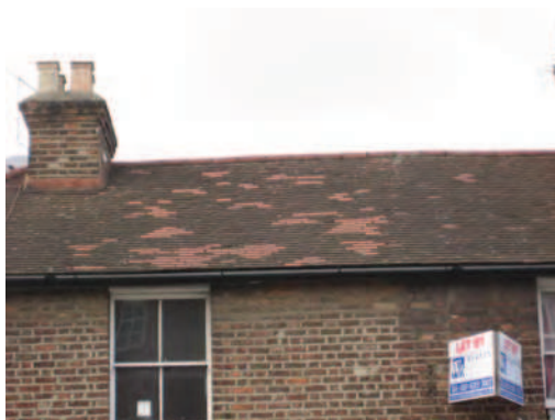
Picture 5.60 One of the six identical chimneystacks containing good clay chimney pots along the Whitchurch Lane terrace (nos. 1-12)
