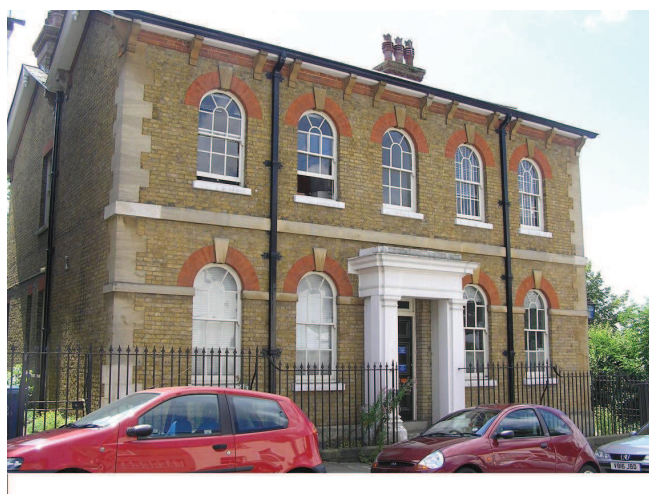
Picture 1.1 Former Police Station, West Street, Harrow on the Hill
