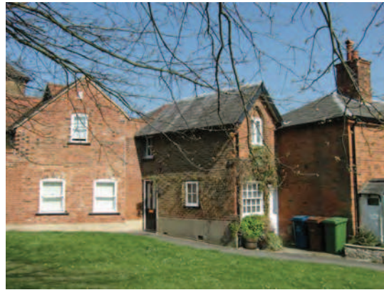
Picture 2.9 No.5 Hill Crest, Green Lane
