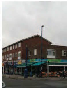
Picture 5.68 Street furniture clutter at the junction of Whitchurch Lane and Edgware High street
