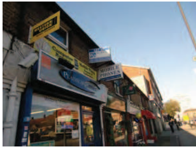
Picture 5.71 Signage cluttering shopfronts on Whitchurch Lane
