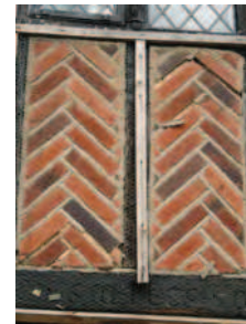
Picture 3.67 Herring bone patterns infilling mock timber framing panels on the locally listed Gate House Lodge, Old Church Lane
