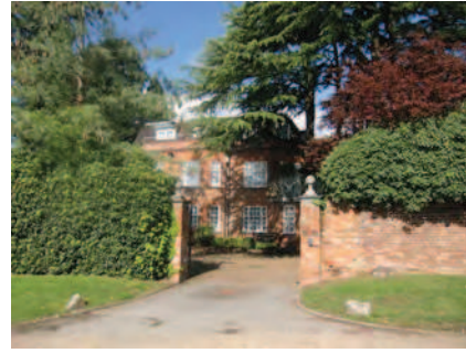
Picture 1.48 Good brick boundary wall to Wellington House
