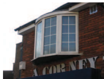
Picture 5.47 Bay window to no. 81 High Street. Although it could benefit from replacement with the use of timber to create more delicate transoms and mullions
