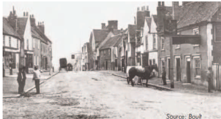
Picture 5.10 View looking south east with the old Masons Arms pub on the right (approximately 1900s). Source: local history library.
