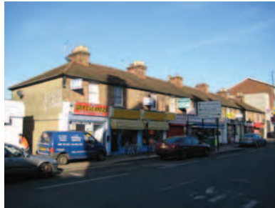
Picture 5.56 Nos. 1-12 Whitchurch Lane. A good Victorian terrace with their original timber sash windows
