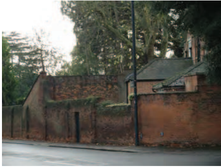
Picture 1.47 Listed wall to Hill House
