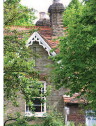
Picture 2.65 Decorative timber bargeboards, and clay ridge tiles and historic timber sash on a property along Stanmore Hill
