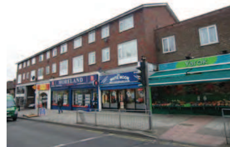
Picture 5.32 Lanson House, Whitchurch Lane offers the opportunity for enhancement
