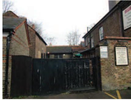
Picture 1.40 Attractive single storey stabling/outbuildings to the Vine
