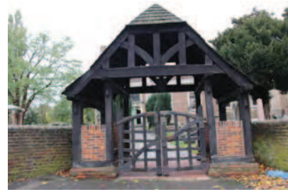
Picture 6.46 Church of St. Lawrence grade II* curtilage listed Lych Gate
