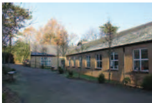
Picture 6.59 1970s Structures
