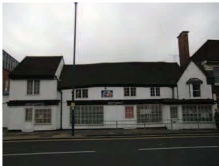
Picture 5.31 Grade II listed nos. 63-67 (odd) High Street, Edgware
