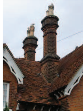
Picture 1.20 Chimney and gable detail of Spring Pond Cottages
