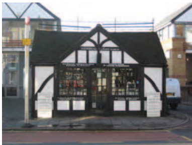
Picture 5.53 The positive unlisted Tudorbethan style no. 103 High Street, Edgware, with good metal railings above
