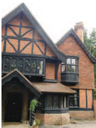
Picture 3.43 Varied roofscapes, decorative mock timber framing, tile hanging and jetty overhang
