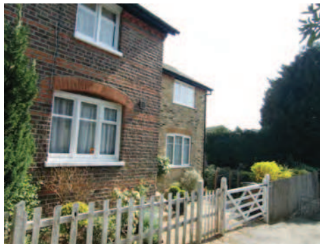
Picture 2.67 Timber casement windows and brick banding detail on Park Cottages on a small side road off Green Lane
