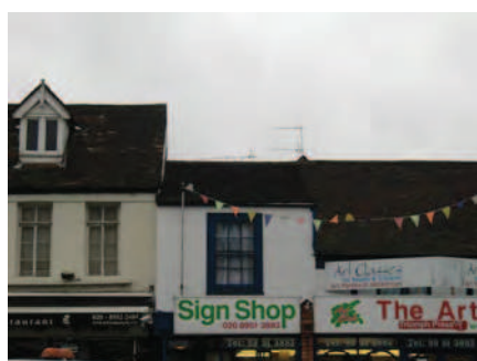
Picture 5.44 Unusual and complex roof structure nos. 89 and 91 High Street, Edgware
