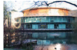
Picture 6.58 Contemporary Structures
