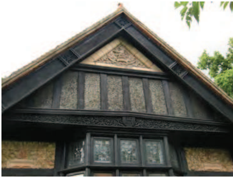
Picture 3.38 Decoratively carved timber work to gable end with delicately carved terracotta panel and stone mullioned windows within
