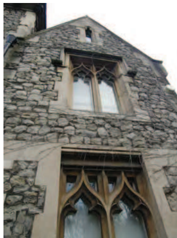
Picture 1.29 Detail of Stanmore Hall - grade II* listed
