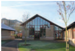
Picture 6.57 Contemporary Structures
