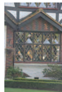
Picture 6.73 Timber/metal leaded light windows
