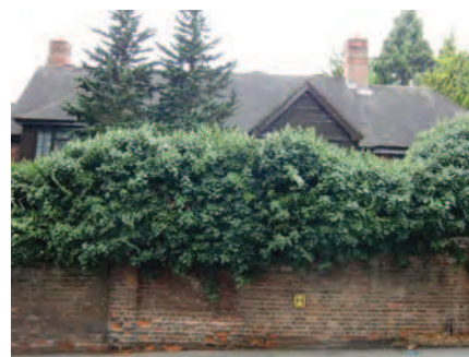
Picture 3.55 Grade II listed wall on Old Church Lane, which provides a good setting to Temple Lodge
