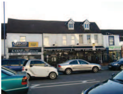
Picture 5.40 No. 85-89 High Street - likely to date to the 18th century with timber framing hidden behind render facing
