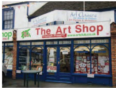
Picture 5.62 Use of modern fascia boards, stall risers and pilasters along Edgware High Street
