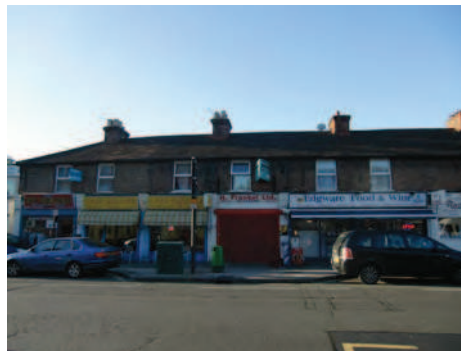
Picture 5.23 Nos. 1-8 of the good Victorian terrace, including shopfronts, along Whitchurch Lane (which goes up to no. 12)
