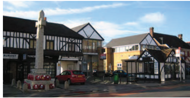
Picture 5.38 Key view towards the grade II listed World War I memorial and the nearby no. 103 High Street, Edgware (the former smithy)
