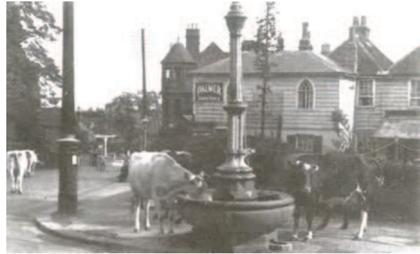
Picture 3.65 The water fountain bowl in its former location on Stanmore Hill in the 19th century
