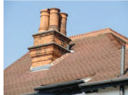
Picture 2.60 Prominent chimney with clay chimney pot, decorative ridge tiles and tile banding detail, Green Lane
