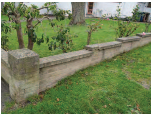
Picture 4.29 Low wall to one front garden along Lower Kerry Avenue
