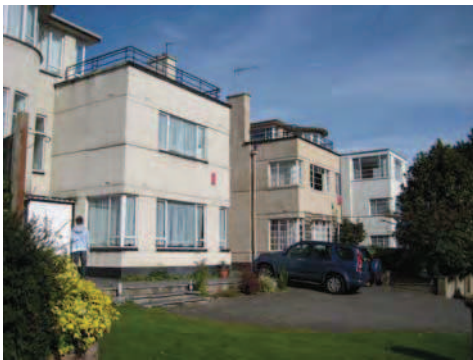
Picture 4.43 Numbers 4 (centre) and 6 (left) Valencia Road, with number 2 in the background
