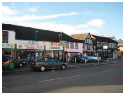
Picture 5.15 View westwards along the High Street illustrating the high density, small scale, linear terraced development that characterises the Conservation Area
