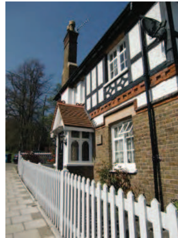
Picture 2.71 Soft picket fencing surrounding the locally listed The Cott, no. 80 Stanmore Hill
