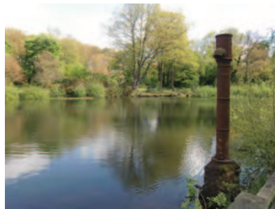
Picture 1.42 Victorian water pump
