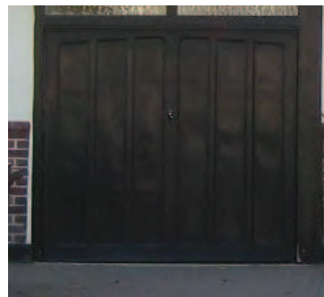
Picture 6.76 Heavy timber pointed garage doors
