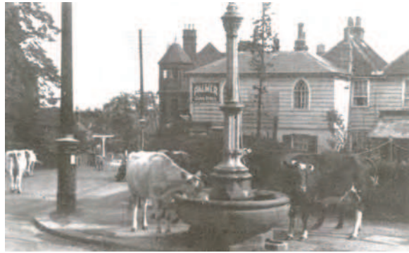
Picture 2.78 Historic cattle trough when it was located in the Stanmore Hill CA, but which is now located in the Old Church Lane CA
