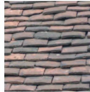
Picture 5.59 Clay tiling on no. 105 High Street - Clay tiling is an important element of historic fabric and detailing that should be retained within the Conservation Area
