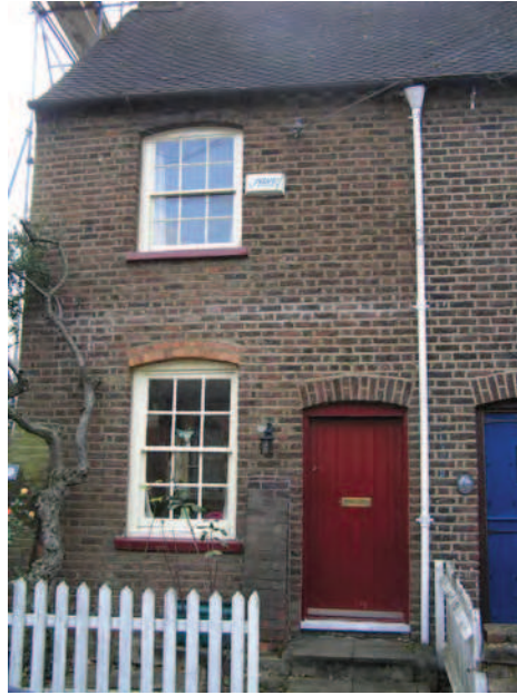
Picture 3.5 29 Middle Road, Harrow on the Hill
