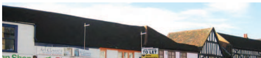
Picture 5.42 View of roovescape along the High Street - the steep pitched clay tiles roofs, with slightly varying heights and roof structures, is one of the most distinctive architectural characteristics of the area
