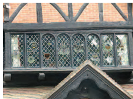
Picture 3.44 Stained glass detail to the leaded light oriel window with delicately carved timber work around it
