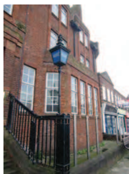
Picture 5.67 Positive unlisted Police Lantern to the Police Station, Whitchurch Lane 326
