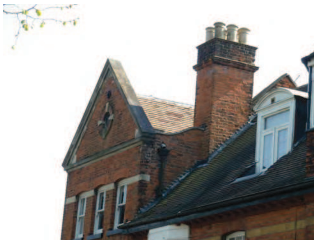
Picture 2.47 Roofscape of locally listed nos. 103 to 107 (odd) Stanmore Hill
