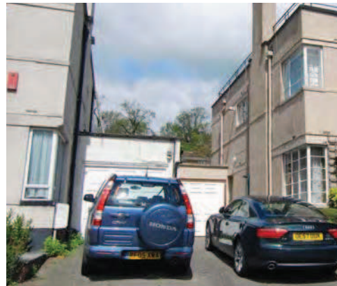
Picture 4.92 Garages between numbers 4 and 6 Valencia Road, number 4 with the original sundeck feature above
