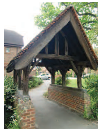
Picture 3.58 Lych gate by Cherry Tree Way on Old Church Lane
